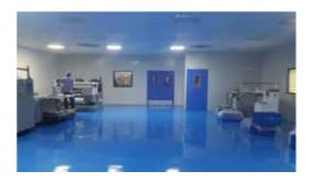
Medical institutions floor needs to be free from allergens and dust. Epoxy acts as a concrete floor sealant. They are safe and easy to clean, preventing microbial growth. The floor coatings of companies manufacturing medicinal drugs should manage to resist most oils, acids, and solvents
