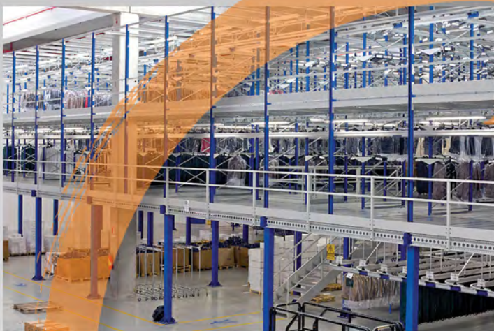
Metal racking and mezzanine floors
