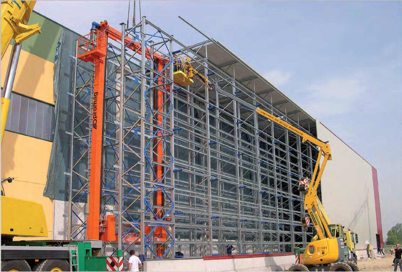
Rack-Supported Buildings (Self-Supported System)
